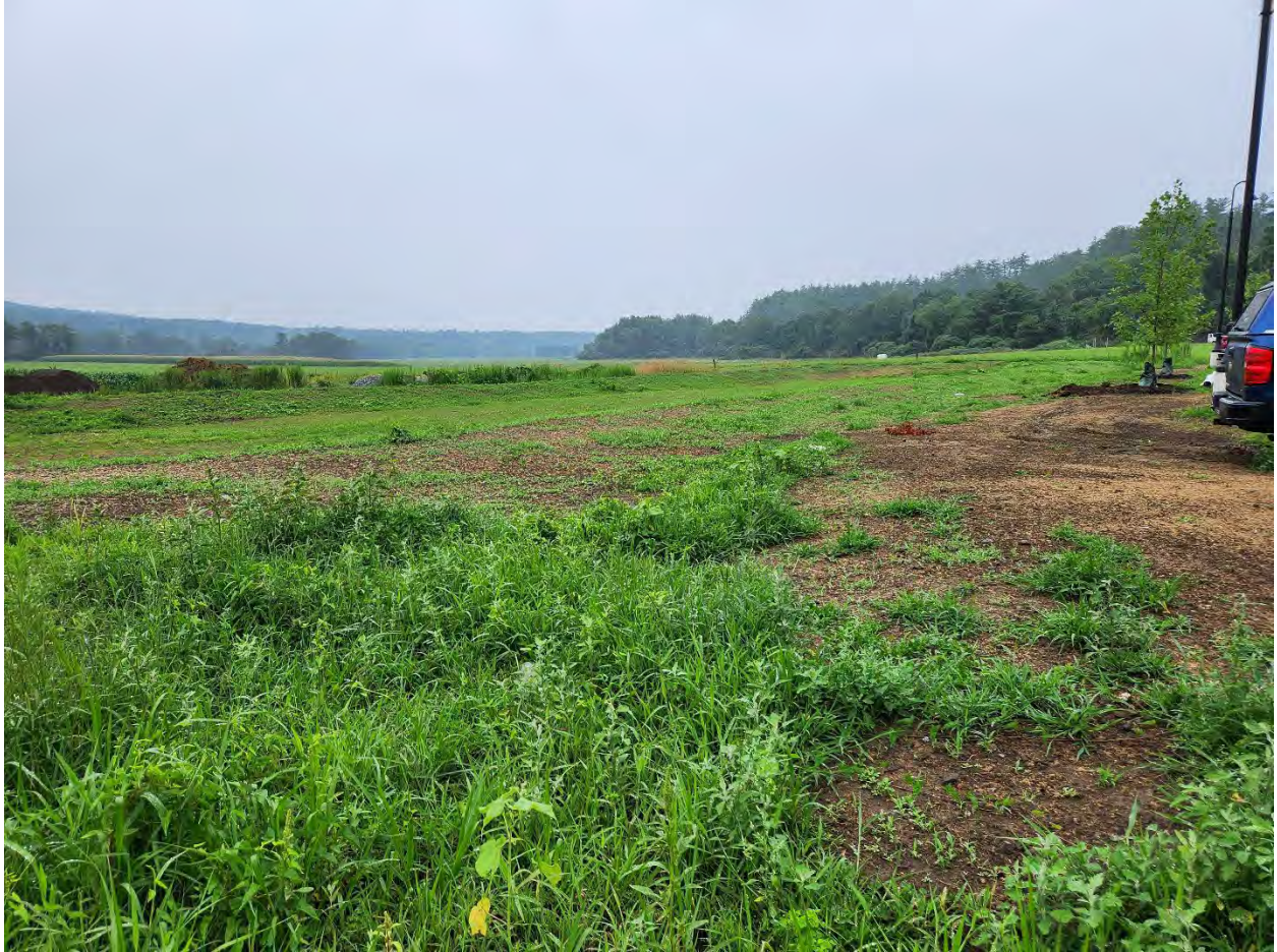
Photo 1a Looking southeast at proposed location of Detention Basin. This is prior to the installation of the outlet structures and spillway. Outlet structure and spillway have been installed (August 2025)
